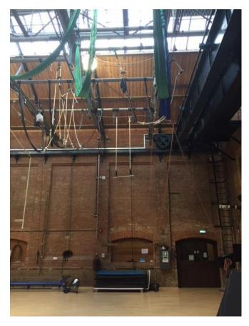
5 pulley systems (3:1), height adjustable rigging points for single-point aerial disciplines.
